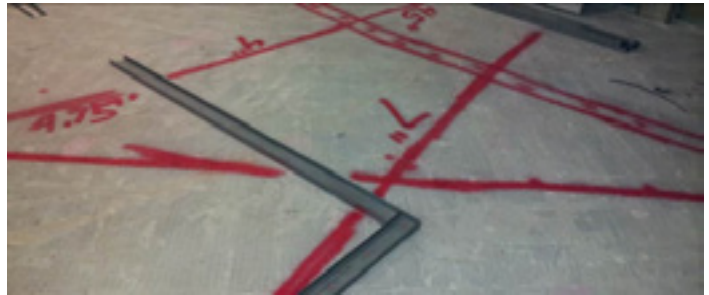
Figure 3: Sample markings identifying electrical utilities in/below concrete with appropriate exclusion zone
