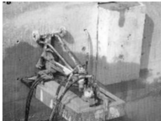
A wire saw could be used to create an opening in concrete instead of a wall saw.
