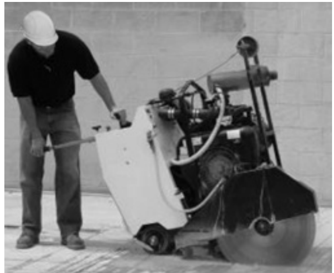
Flat saw making a cut.
