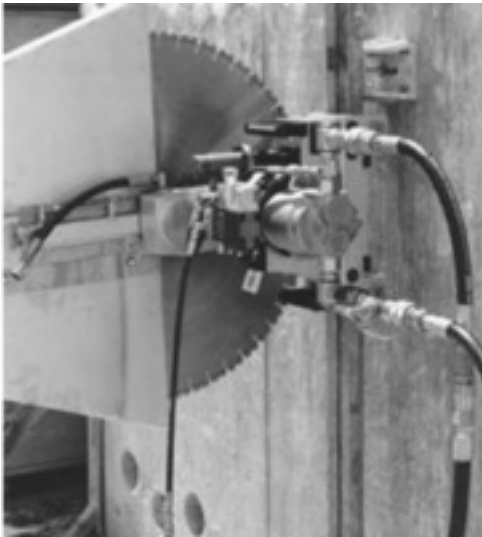
Wall saw preparing to make a cut.
